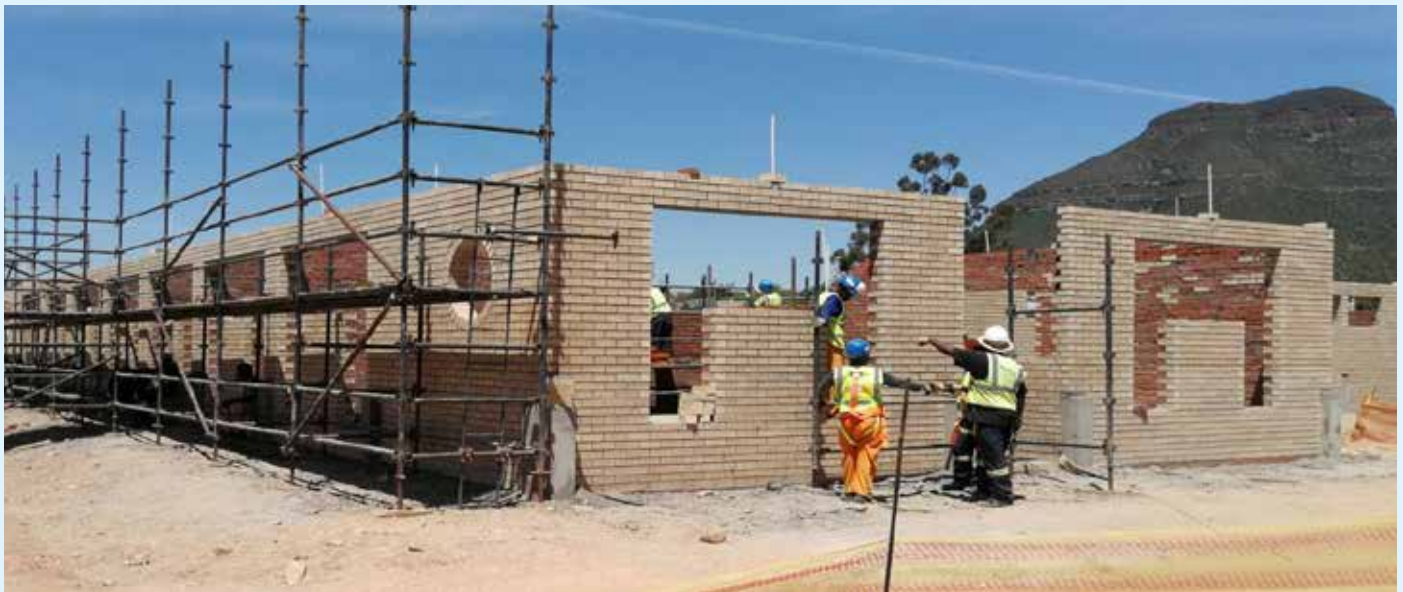
Ongoing construction at Ikhala TVET College Sterkspruit Campus in Eastern Cape
